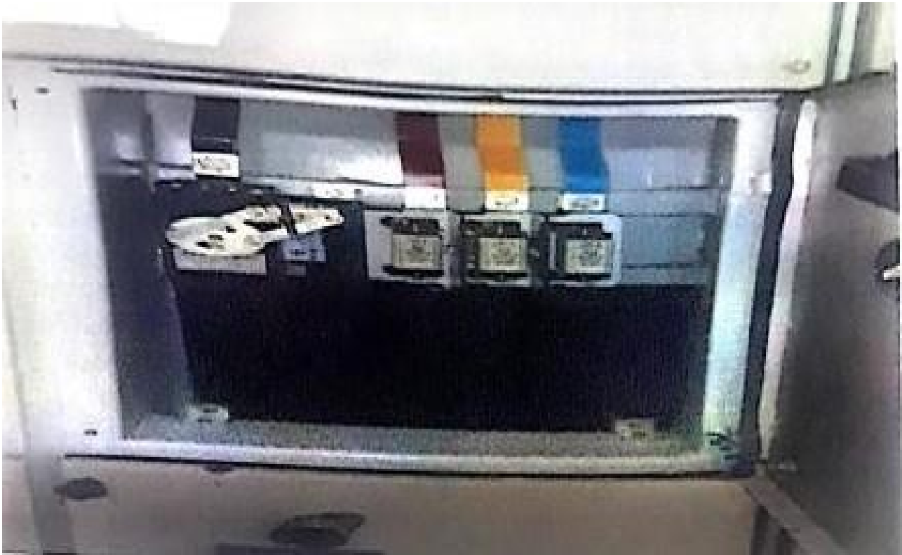
(c) Incomer Panel and Distribution Board for street lighting
