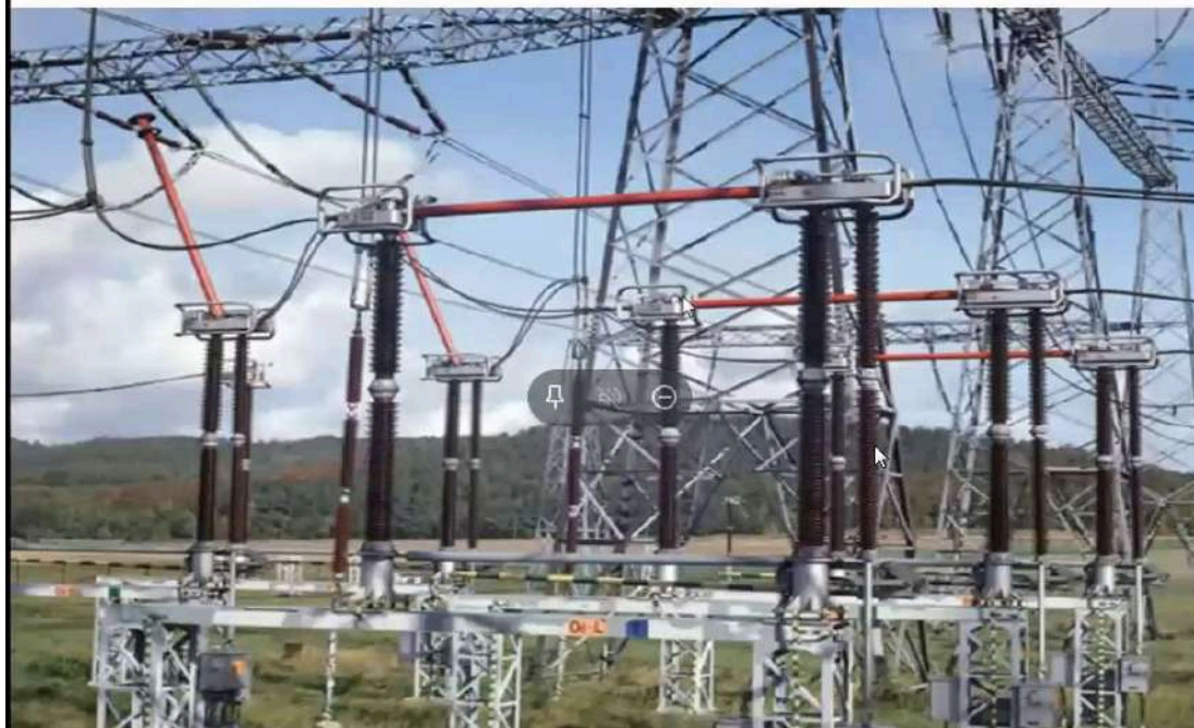
VERTICAL BREAK ISOLATOR IN CLOSED POSITION
